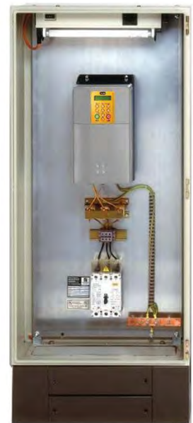
DC590+ DRV equivalent illustrating panel space saving
